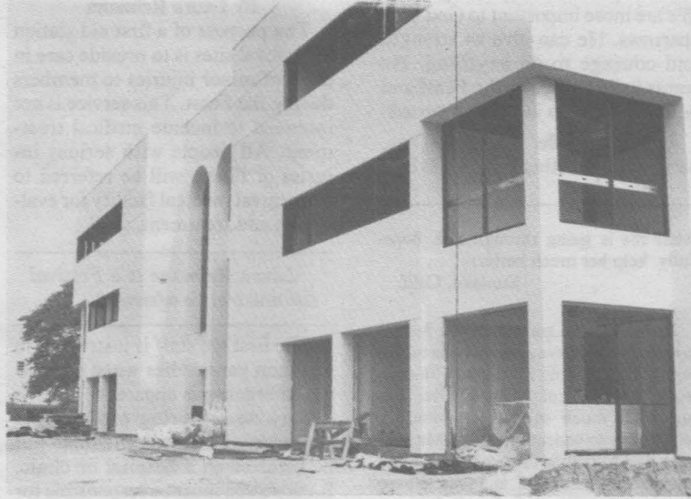
FINISHING TOUCHES —The scaffolding removed, most of the exterior work on the College Administration Building is complete.
